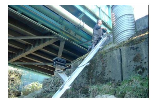
Photo 3. Placement of one of two DIDSON sonars and ramp upstream of the 5<sup>th</sup> Street bridge
