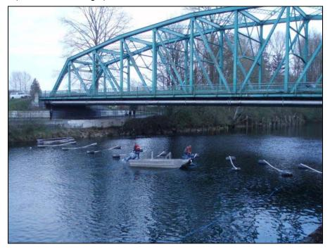
**Photo 2.** Placement of the 3-cable array upstream of the 5<sup>th</sup> Street bridge prior to anchoring, April 2008. Photo looking downstream from west to east shore (river right to river left).
