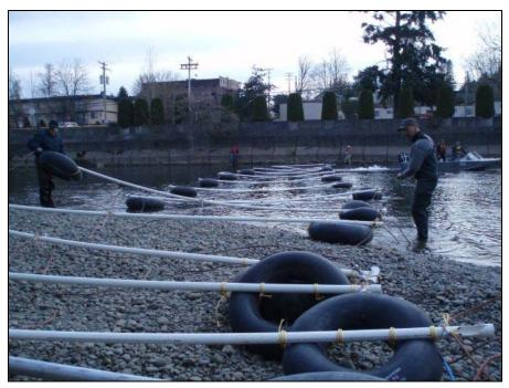
**Photo 1.** Assembling and installing the 3-cable array, April 2008. Photo looking from east to west shore (river left to river right) at low tide.
